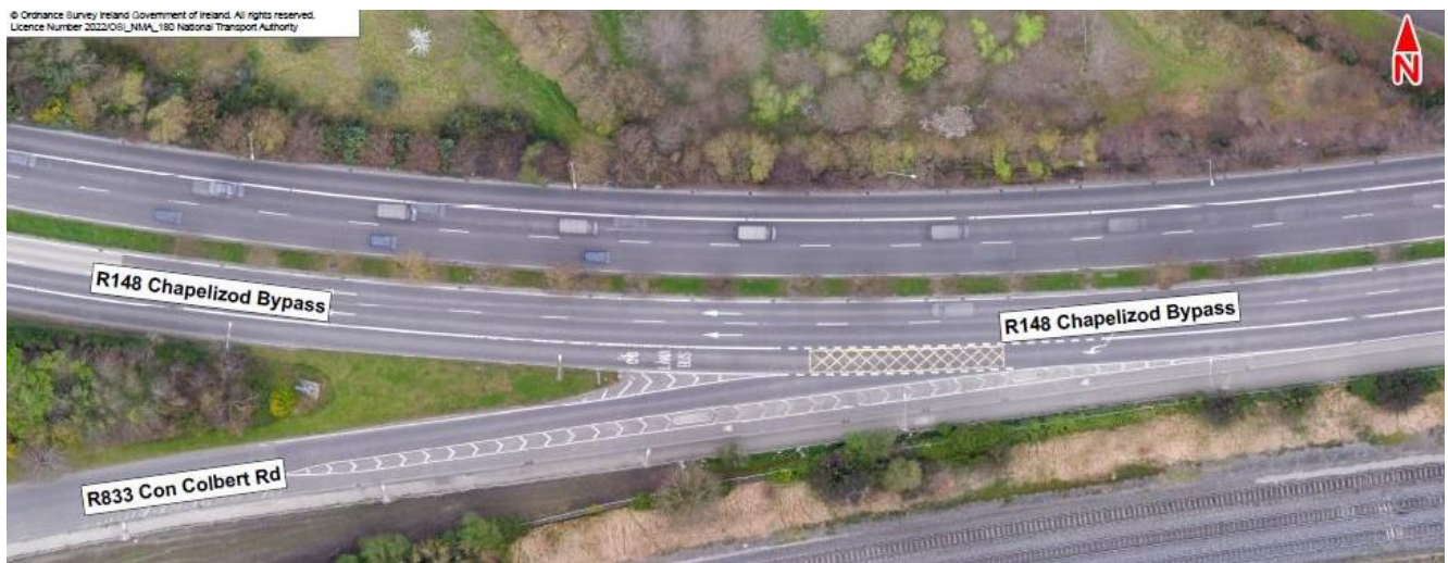
Image 5.21: R833 Con Colbert Road Junction (East)
