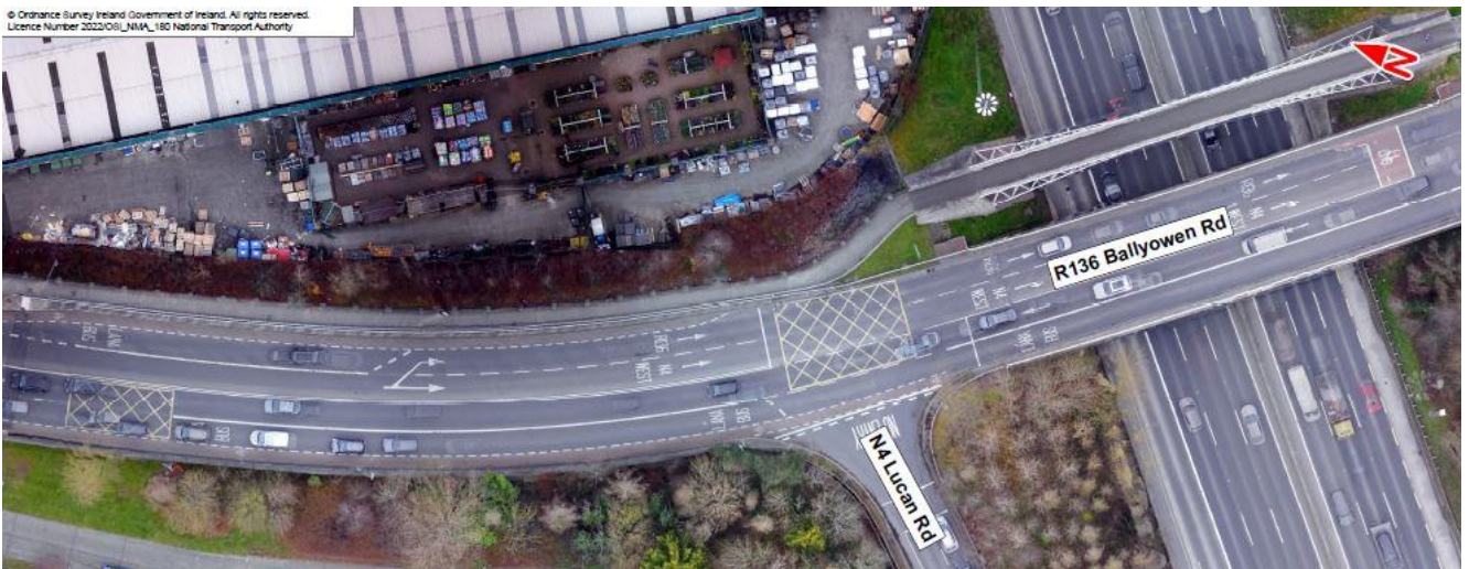
Image 5.3 R136 Ballyowen Road / N4 eastbound off-slip road Junction
