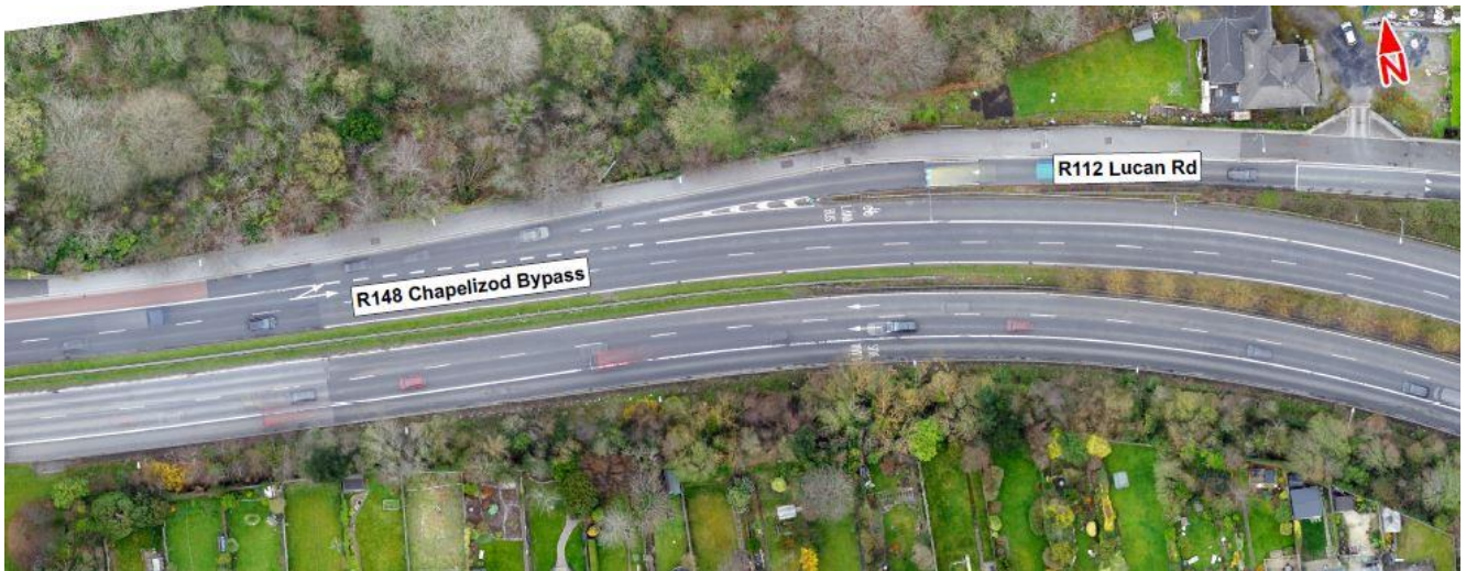
Image 5.18 R148 Chapelizod Bypass / R112 Lucan Road Junction
