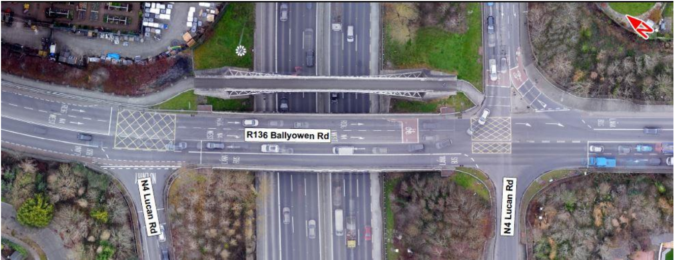
Image 5.2 R136 Ballyowen Road / N4 westbound on / off-slip roads Junction
